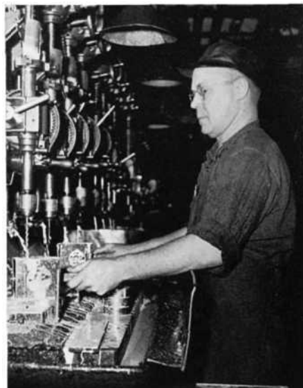
Charles F. Phelps of 1-8 topped the list of Cash Awards of award winners with a $35.00 prize for a constructive suggestion, covering the use of a second jig in the drilling operation on round dies, thereby resulting in increased production.
