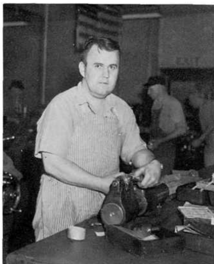
HAROLD A. DORAN , 2-52, won a $50.00 cash award for his Suggestion for installing markings on supermikes which allows O.D. Grinder to know when he is near low grinding limit.
